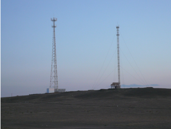
Plate 38 Panels of solar cells (at the bottom of antenna) for a transmission station near Fuyun
